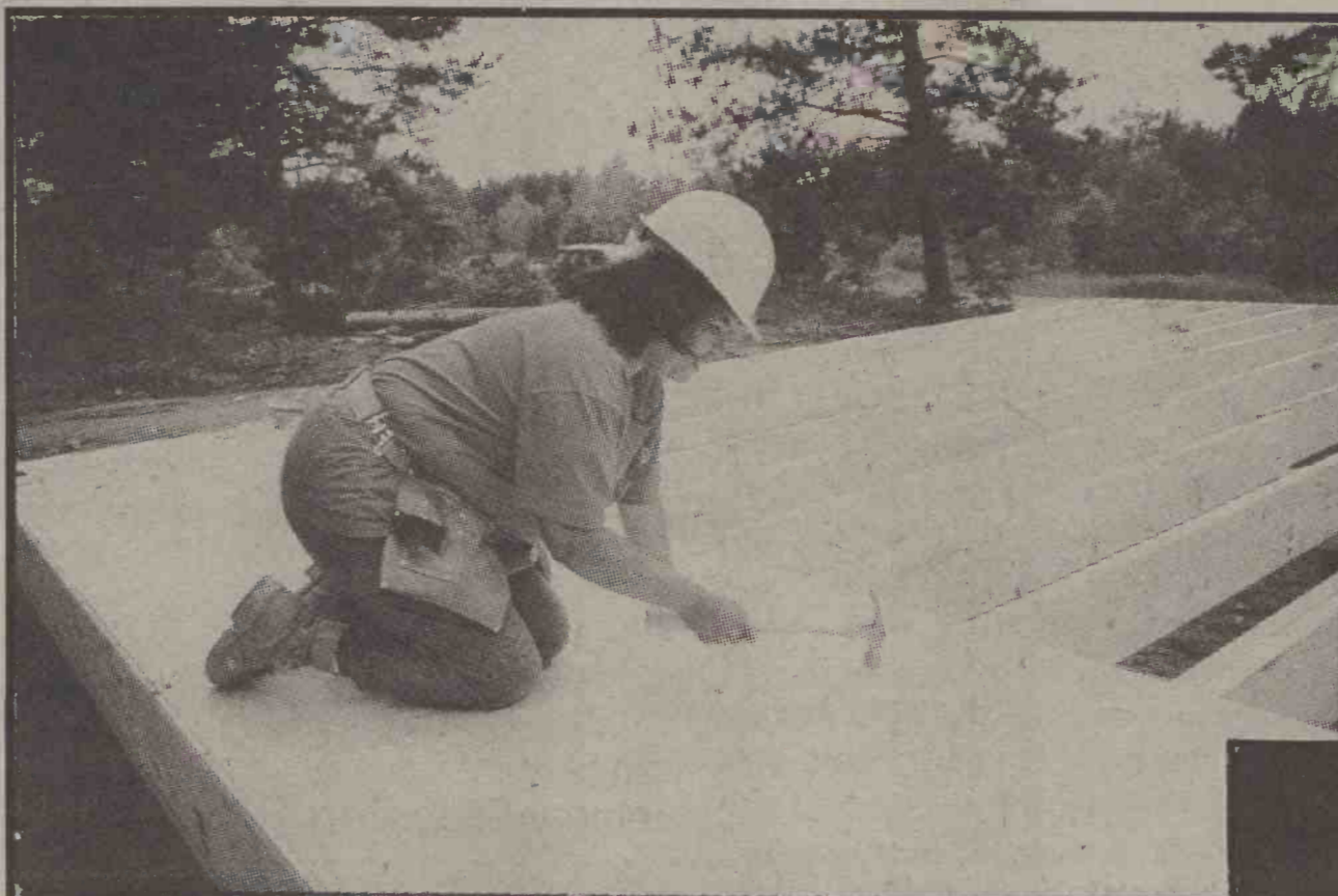
Linda Niganobe installs the subfloor on the house that will be hers upon completion
