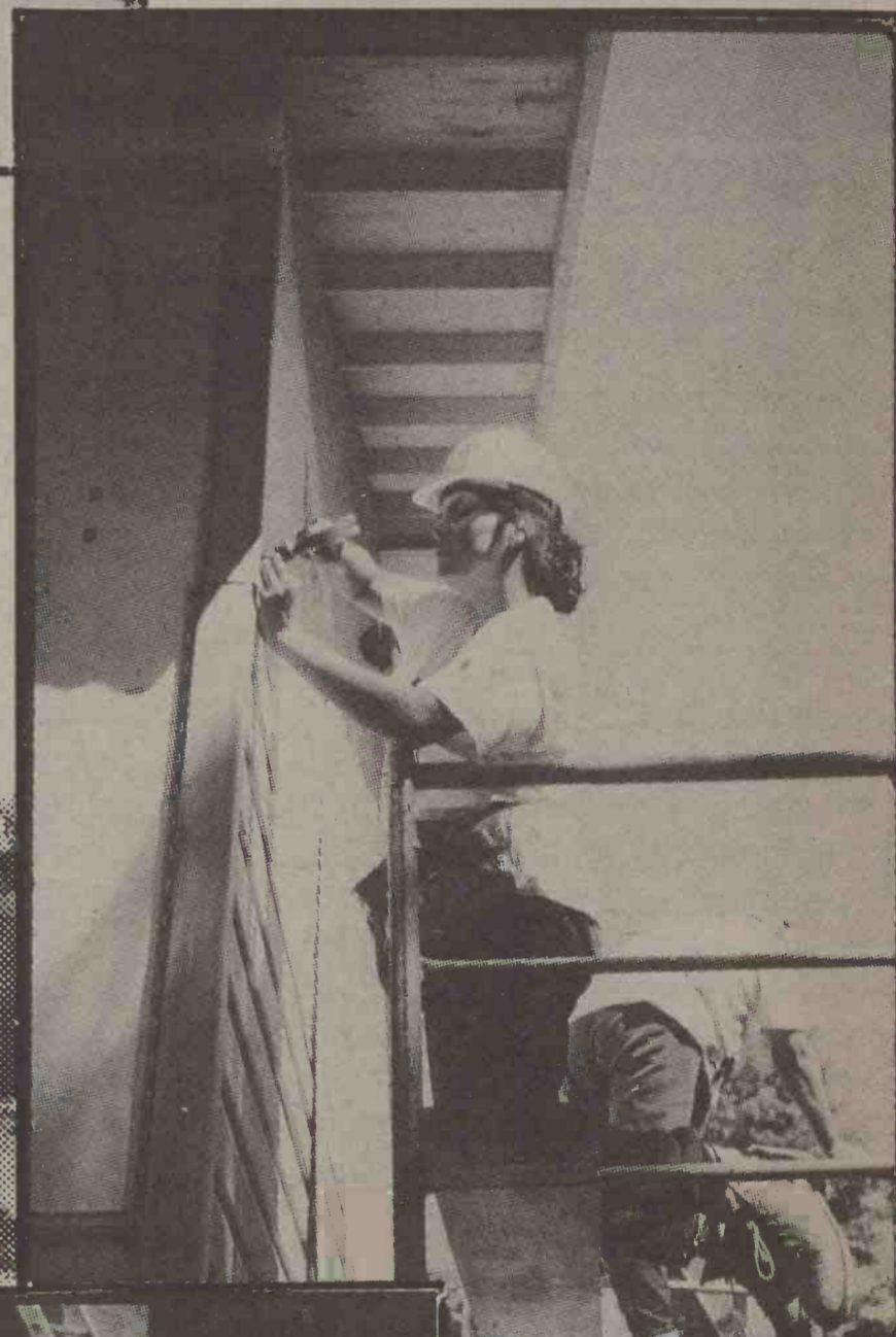
Janice Boyer installing siding on house exterior.
